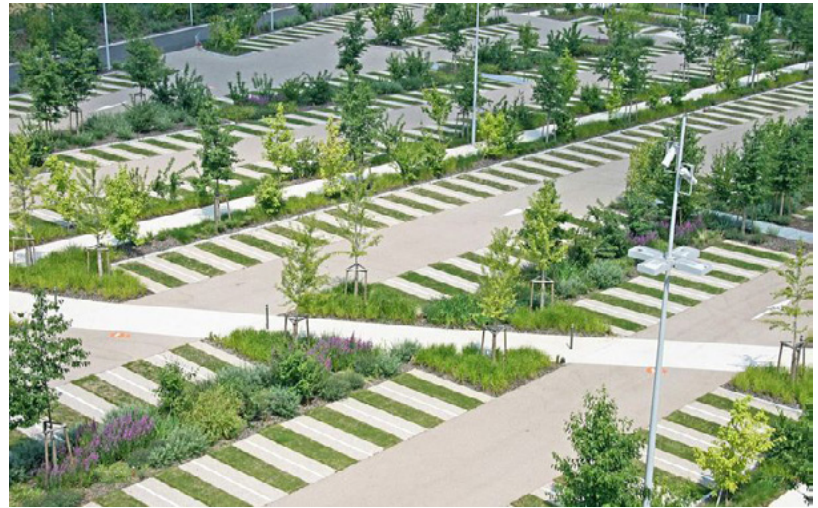
A parking garden with bioswale plantings helps capture stormwater for a large area of impermeable parking surfaces.
